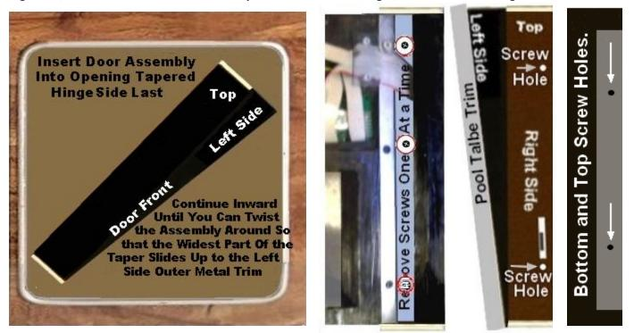
Install a 1 & 1/8 inch Door Lock in New Door. Insert the Door Assembly Into the Opening, The Right Side of Door Assembly First. Continue Inward Until YOU can Twist the Assembly Around So the Assembly Can be Pulled forward Widest Part of Tapered Side Toward the Top and Up against the Table Trim, the Right Side Bottom in Also in Contact with the Trim. Open the Door and On the Left Side Remove the Center Wood Screw Holding the Hinge to the Assy...
